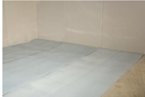
Lay the Elastic mat on top of the sheeting with the adhesive layer and protective foil facing upwards. Obviously these must not overlap.
