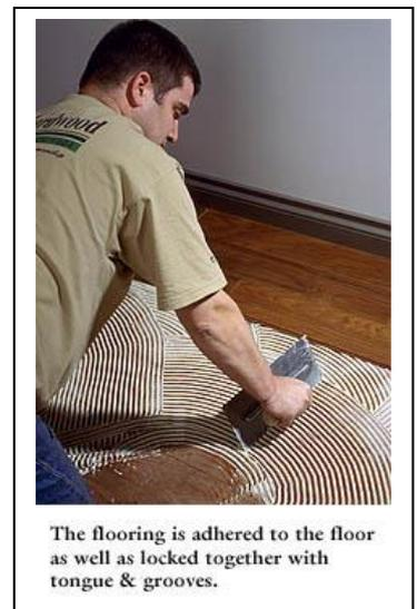
The flooring is adhered to the floor as well as locked together with tongue & grooves.
